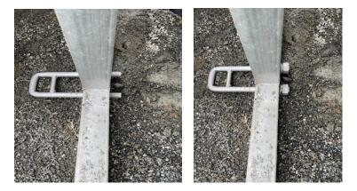
STEP 2: Attach 2 nuts to the bolt threads
