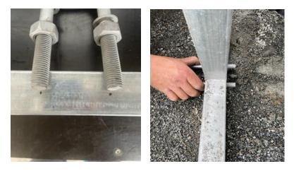
**STEP 1:** Mark and drill 2 x 20mm holes through the bottom rail in desired position, then place the Anchor Bolt through the holes
