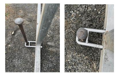
STEP 3: Drive pin into the ground
